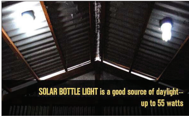
Figure 5.5 Sample of an installed solar bottle (How to Magazine, 2011)
